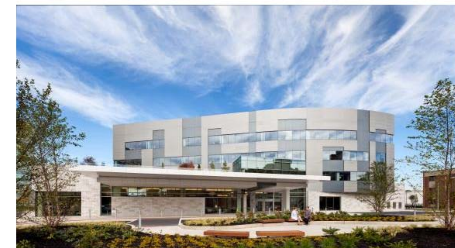
The MD Anderson Cancer Center at Cooper is situated in a previously developed urban site, a former parking lot. The building's south facade, shown here, combines metal panels, natural stone, and high-performing insulated glass. The main entry is accessed via a shared vehicular drive around a landscaped plaza. A two-story section with a raised healing garden on its canopy roof creates a transition between the four-story building and the entry plaza. Photo: ©Chris Cooper Image 1 of 5
