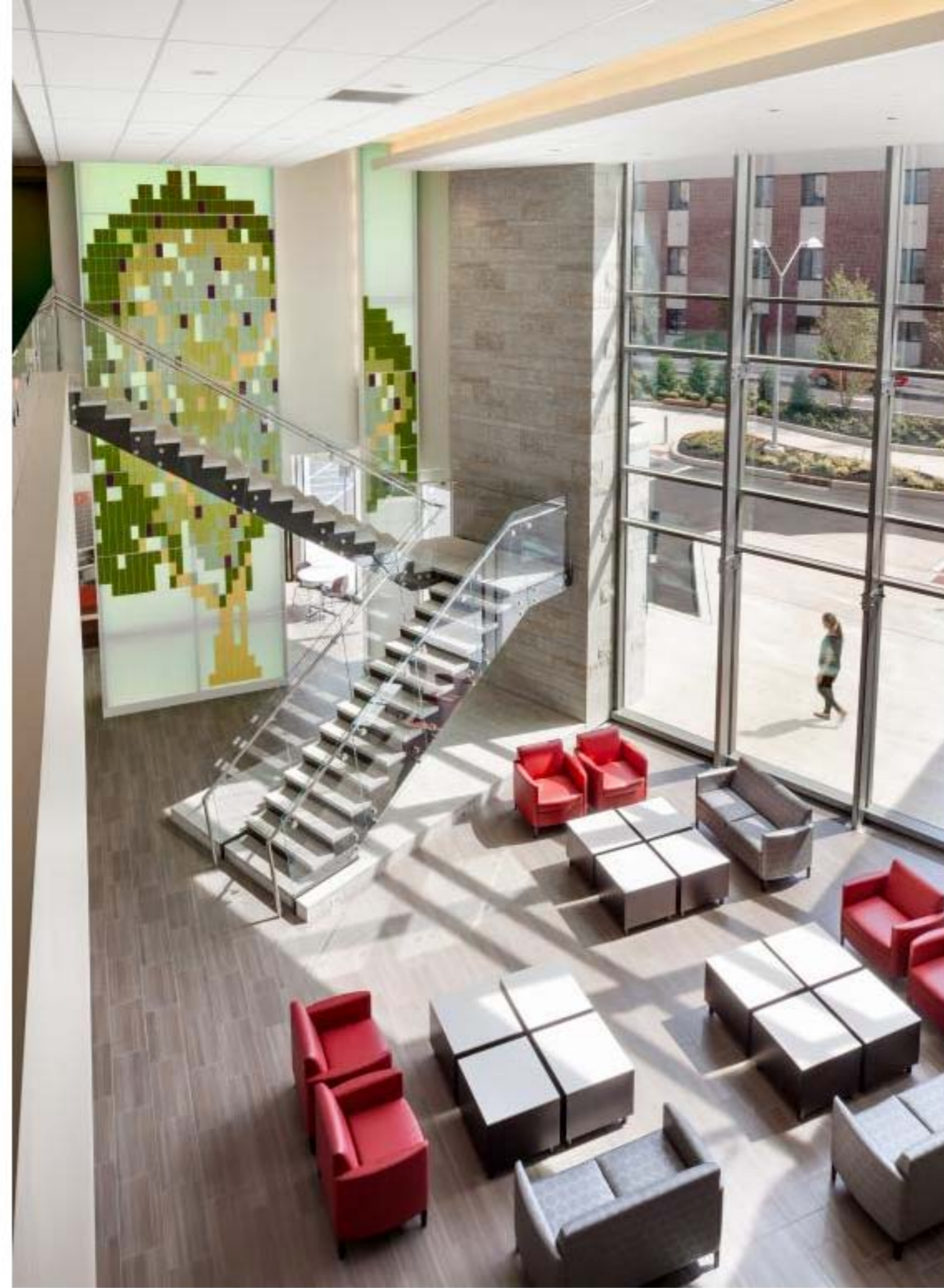
The focal point of the lobby, the Tree of Life is a dramatic two-story sculptural representation. It's made of acrylic panels of different sizes and thicknesses that are evenly backlit with color-changing LED lights. It provides a backdrop for the lobby stairway, which is made of blackened steel and point-supported glass. Photo: ©Chris Cooper Image 2 of 5
